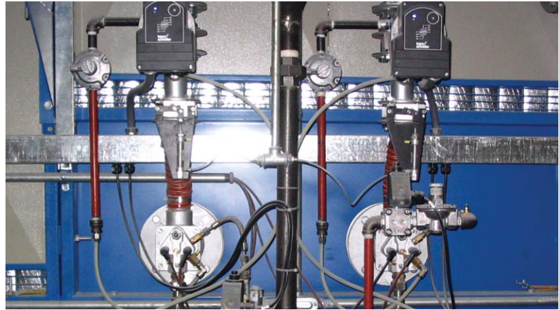
Each burner features a continuous internal pilot with a spark and sense electrode.
