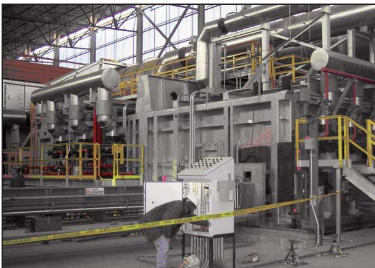
Figure 1 - Nucor Auburn pusher furnace
